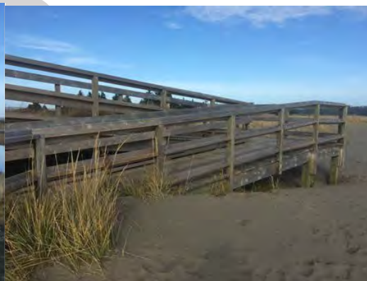
Figure 5: Sand encroaching on boardwalk.
