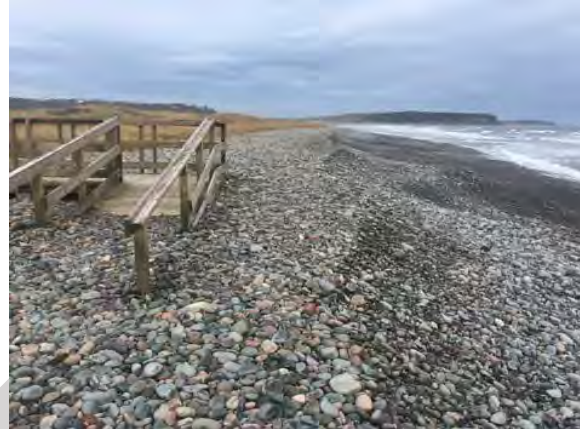
Figure 17: Cobble stones washed up the steep beach face and onto existing boardwalk access.
