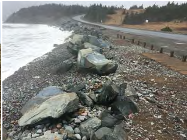
Figure 9: The armour stone near Surfers Parking Lot is showing signs of failure.
