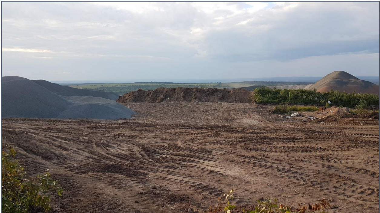
Figure 3. Panoramic view of work areas at Westchester Quarry, facing north, September 1, 2017.
