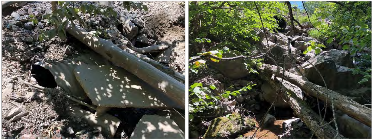
Figure 4. Fish barriers along unnamed stream 1. Top left photo , downstream end of culvert below Westchester Road, a hanging culvert 1+ m above the streambed. Top right photo , a steeply sloped rock waterfall in upper reaches of unnamed stream 1 (above Westchester Road). Bottom left photo , upstream end of the hanging culvert positioned under the Westchester quarry access road; it was partially blocked by sediment during both survey days. Bottom right photo , downstream end of the quarry access road culvert, which was 2+ m above the streambed. July 13, 2022.
