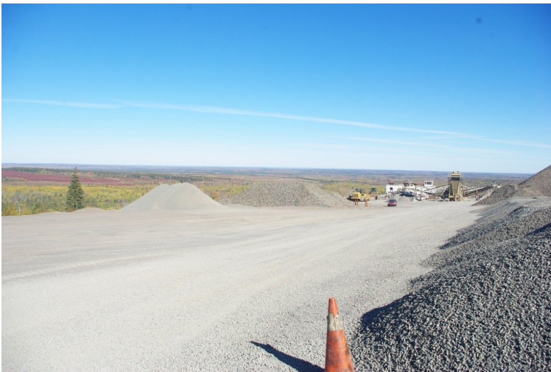
Photograph #1 View of the Crushed Stone Stockpile Area (facing northeast)
