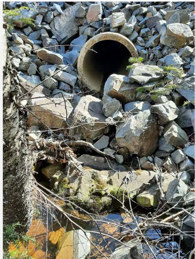
Photo 45: Culvert outlet (quarry access road)
