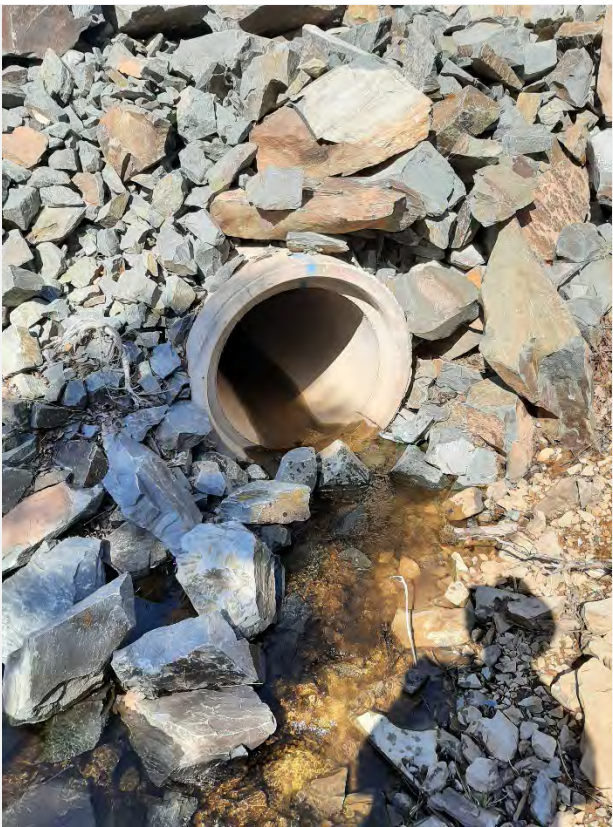
Photo 44: Culvert inlet (quarry access road).
