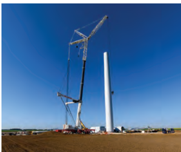
Building the tower
