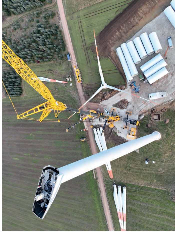
Dismantling wind farm
