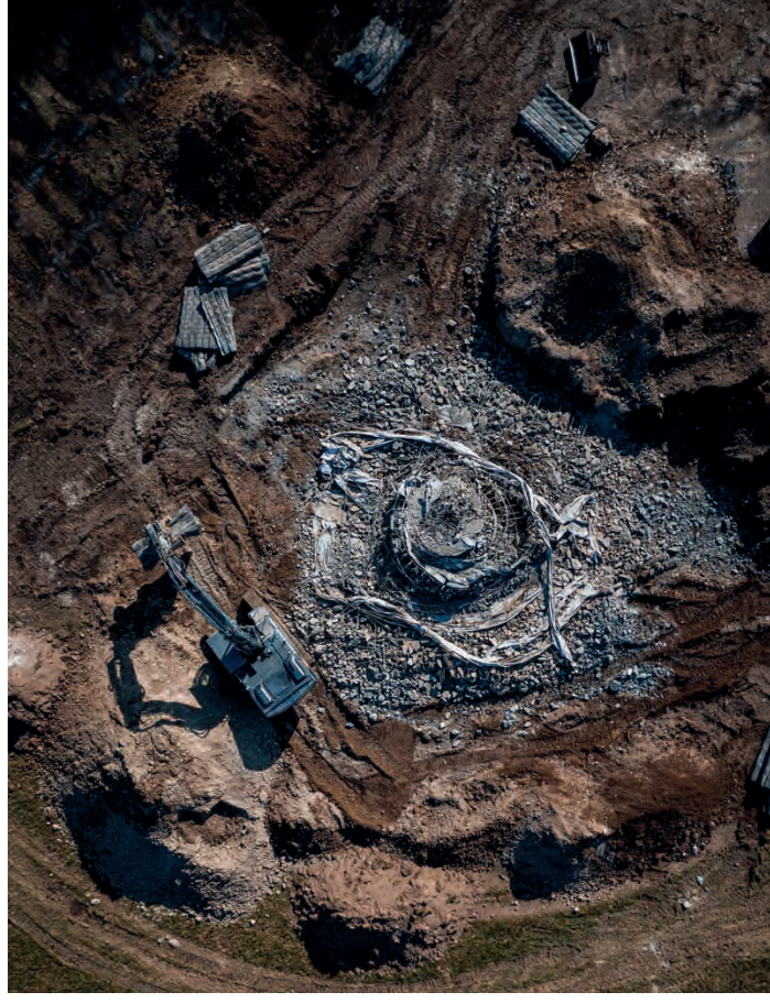
Deconstruction of foundation
