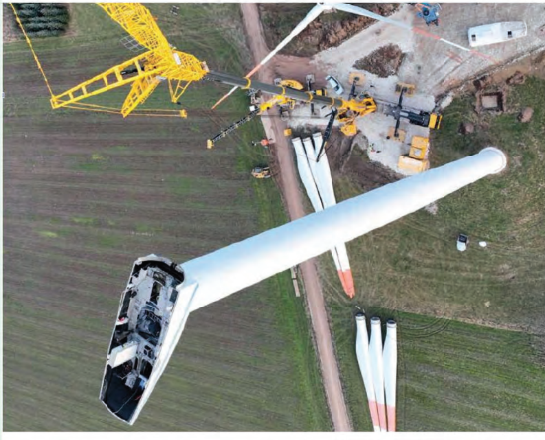
Dismantling a wind farm
