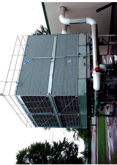
Cooling towers are required to reduce high summer water flows. This will in turn reduce the total effluent flow.
