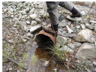
Roadside drainage ditch with culverts under existing quarry access road.
