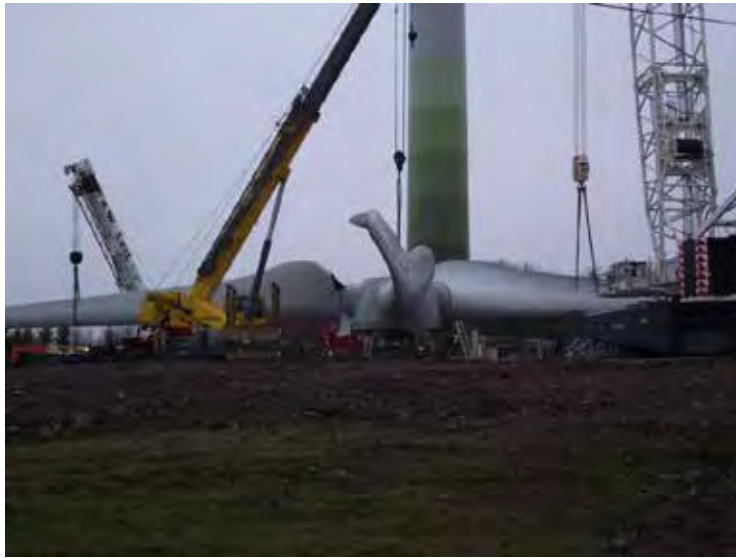
Photo 8. Hub and Blade Lift.
