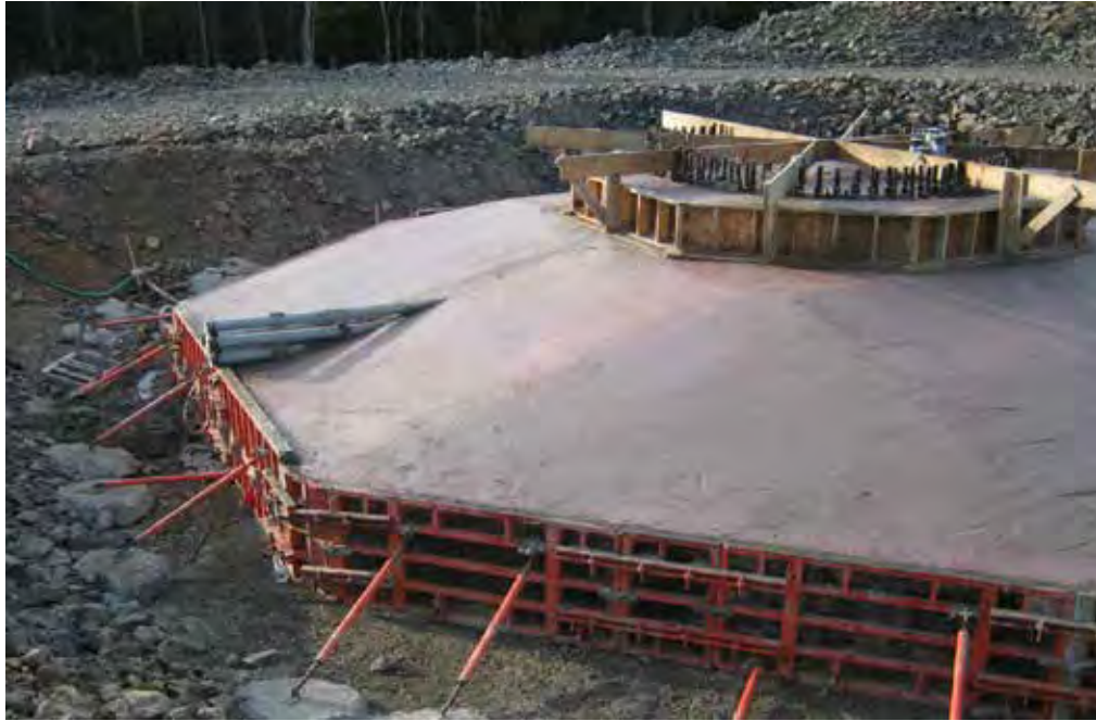
Photo 5. Typical turbine spread footing foundation following concrete pour. Note blasted rock from foundation used on site.
