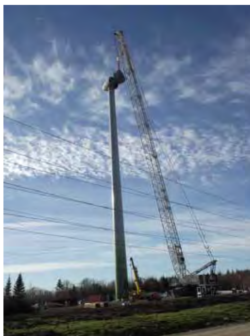
Photo 7. Nacelle Installation
