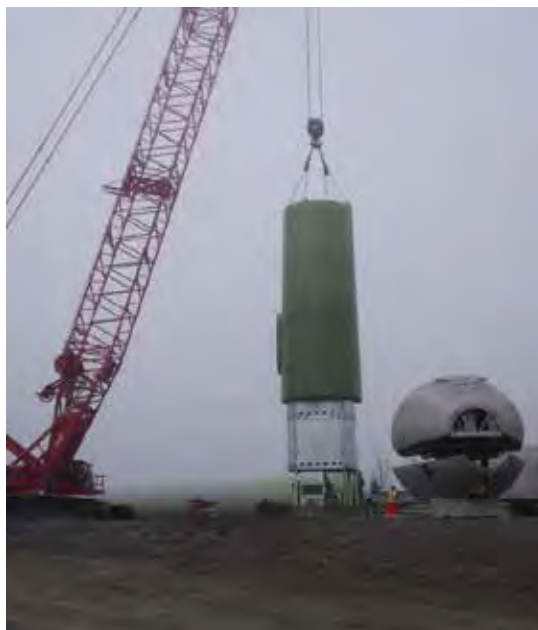
Photo 6. Tower section installation
