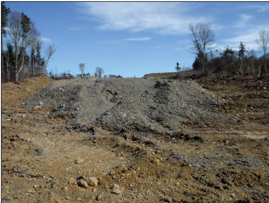
Plate 4: The beginning of the newly built access road looking southeast. Note the grey gravel fill on top of the native orange/brown soil.
