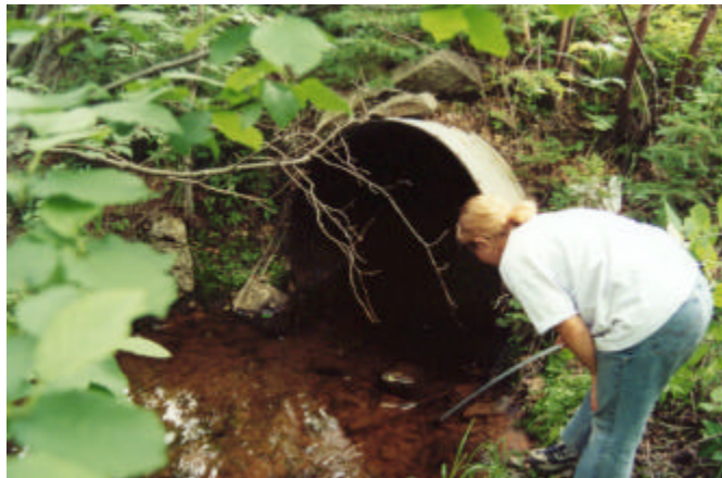
Photo 5 Culvert Directing Stream A Underneath Bear Island Road
