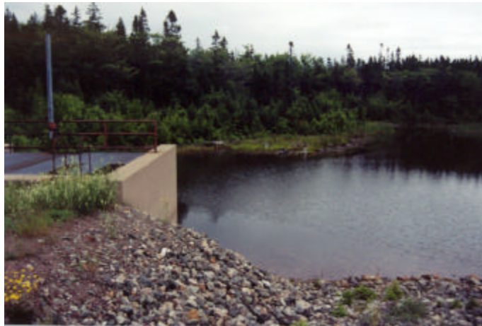
Photo 7 Retention Pond on Stream A
