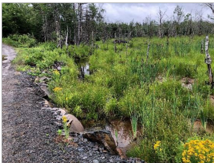
Figure 15. Unnamed tributary 1 of Barren Meadow Brook along the east boundary of the study site, looking upstream of the quarry access road culvert towards the beaver-flooded wetland, July 6, 2022.
