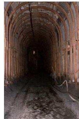
Donkin Mine Tunnel
