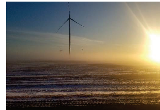
Golden South Wind Project, Saskatchewan
