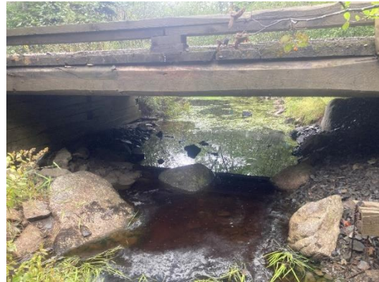
Photo 4: Evidence of open-bottom bridge along WC2.
