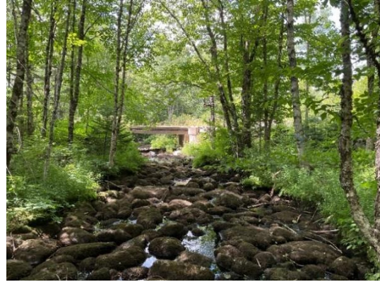
Photo 2: Evidence of open-bottom bridge along WC1.
