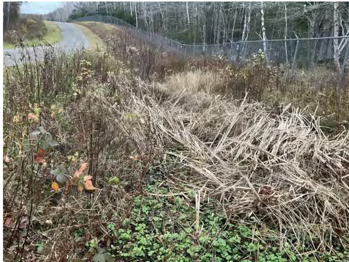
Photo 7: WC7 flowing towards WC8 in LLWU ditch (WC7 and WC8 merge and flow underneath the LLWU access road via culvert towards Landrie Lake)
