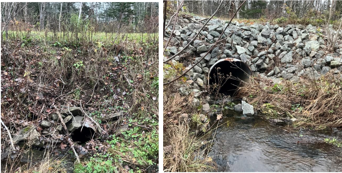
Figure 19: Watercourse crossings along the LLWU access road right-of-way and the raw freshwater pipeline. WC7 and WC8 join (via ditching) and flow through a metal culvert (left), while WC10 flows through a separate culvert (right).
