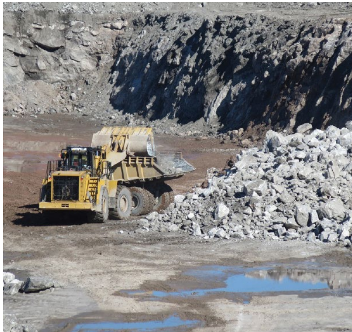
Photo.B.1.2 A 12-yard loader loading a 70-ton truck with gypsum to be hauled to the crusher
