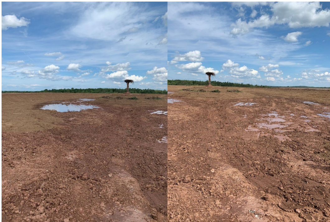
Photo B.2.4 Photos of the pond in the process of being reclaimed. Material was distributed to create a natural catchment area for water, to eventually allow revegetation. A tree was installed with the roots up to provide habitat for Bald Eagle.
