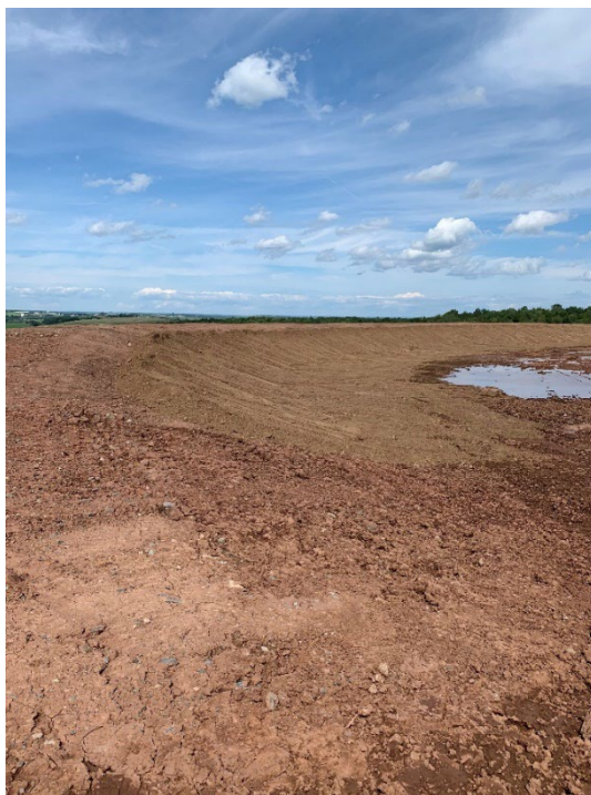
Photo B.2.3 The berm of the pond in the process of being shaped, as material was redistributed to hold water.
