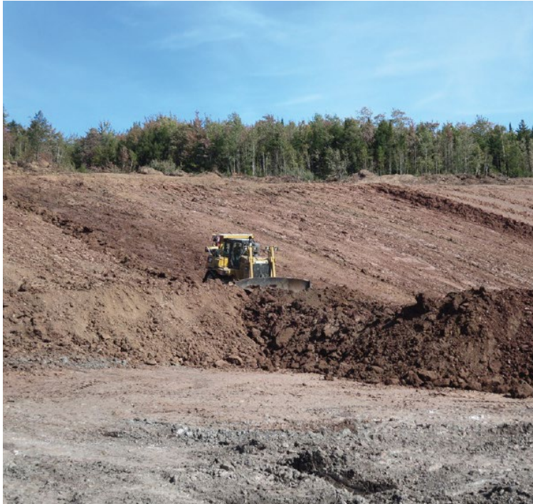
Photo.B.1.6 Bulldozer pushing mud down to uncover gypsum rock.
