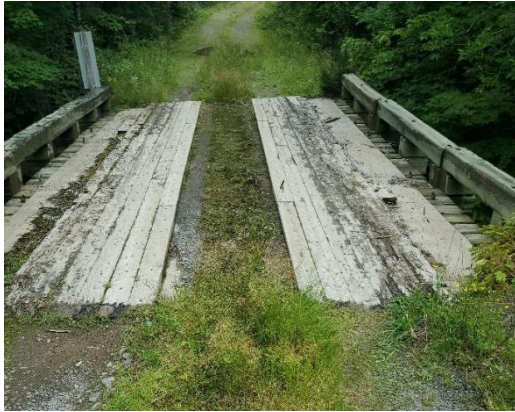
Photo 18. Evidence of a bridge along WC11.
