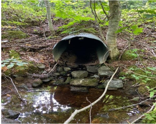
Photo 7. Evidence of a culvert along WC4.
