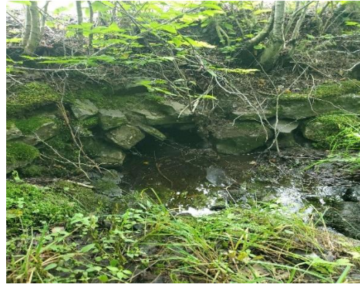
Photo 25. Evidence of a culvert along WC16.
