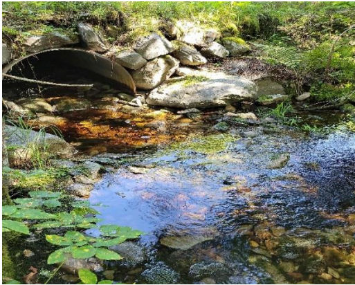
Photo 42. Evidence of a culvert along WC28.
