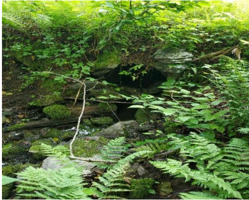
Photo 12. Evidence of a culvert along WC8.
