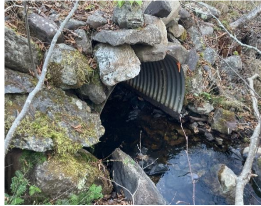
Photo 48. Evidence of a culvert along WC33.
