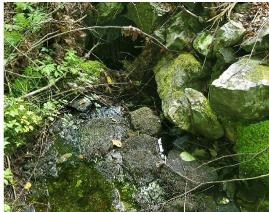
Photo 27. Evidence of a culvert along WC17.
