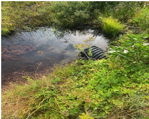
Photo 9. Evidence of a culvert along WC5.
