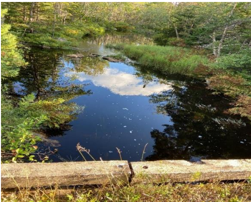
Photo 52. Evidence of a bridge along WC36.
