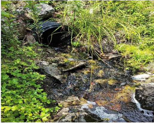
Photo 58. Evidence of a culvert along WC39.
