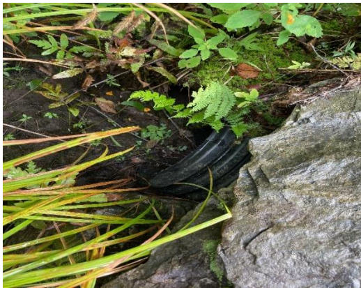
Photo 14. Evidence of a culvert along WC9.
