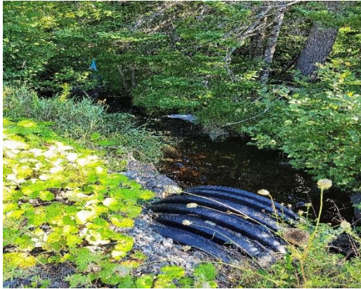
Photo 50. Evidence of a culvert along WC35.
