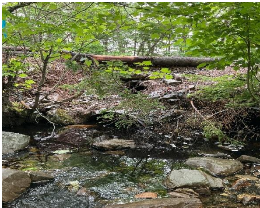
Photo 37. Evidence of a culvert along WC24.
