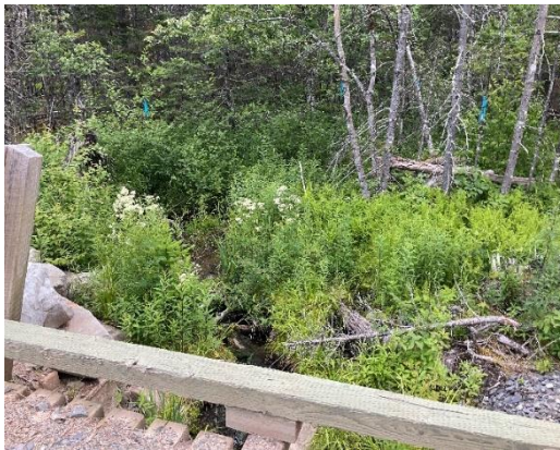
Photo 54. Evidence of a bridge along WC37.
