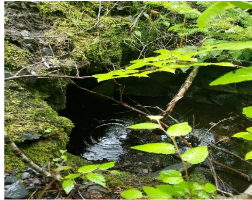
Photo 21. Evidence of a culvert along WC13.
