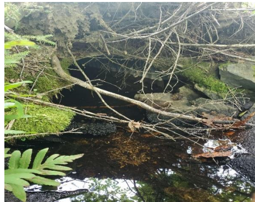
Photo 29. Evidence of a culvert along WC18.
