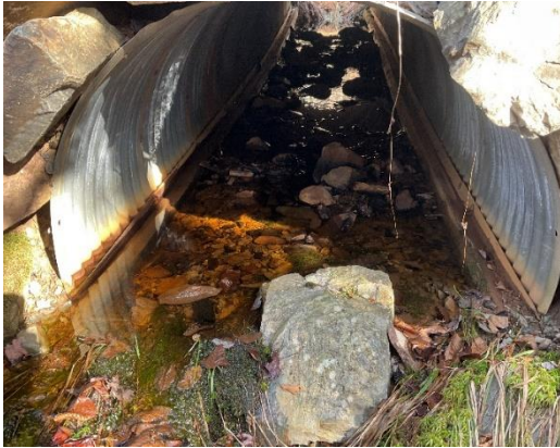
Photo 35. Evidence of a culvert along WC23.
