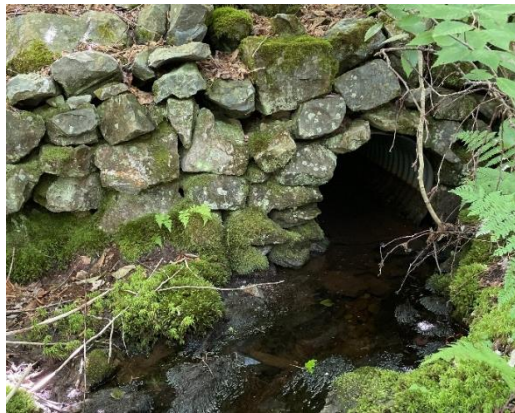
Photo 4. Evidence of a culvert along WC2.
