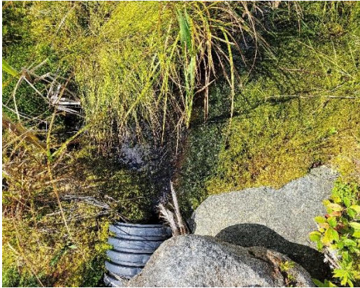
Photo 56. Evidence of a culvert along WC38.
