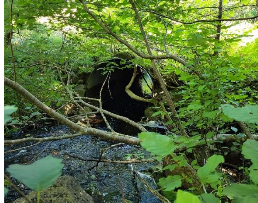
Photo 46. Evidence of a culvert along WC32.
