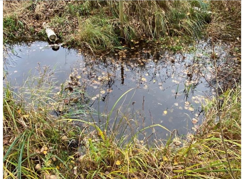
Photo 14: Agricultural drainage culvert (Coleman Brook)
