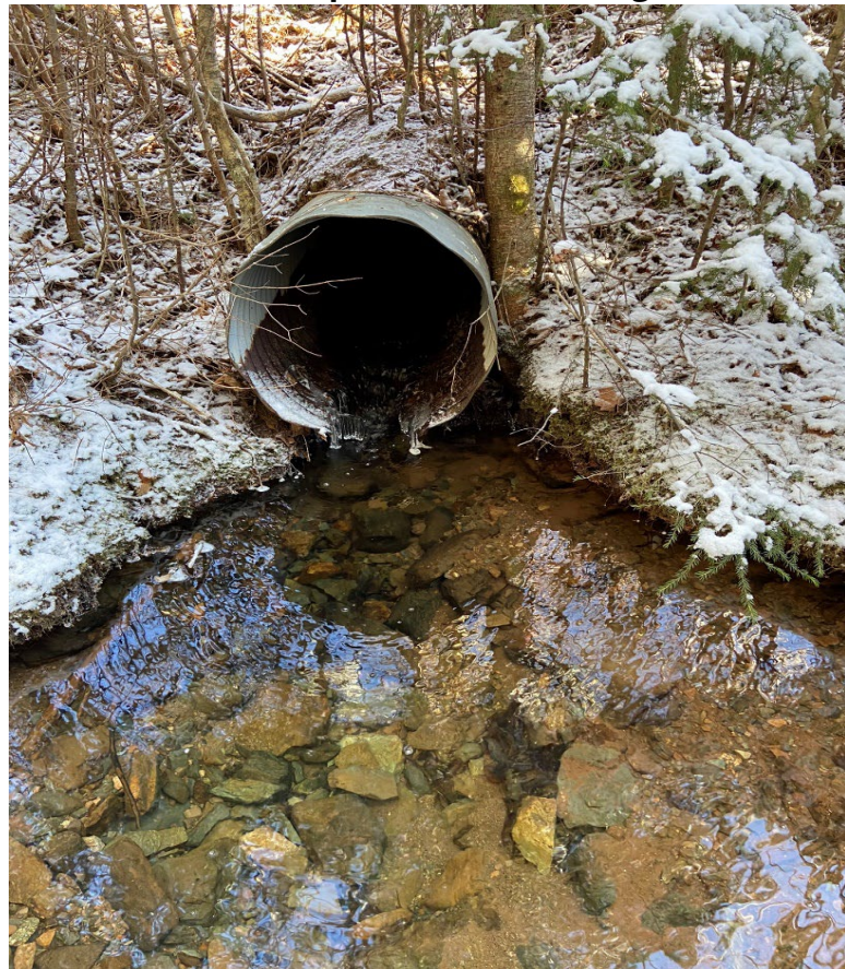
Photo 3: Feature 1 (Culvert at crossing with angular cobble)
