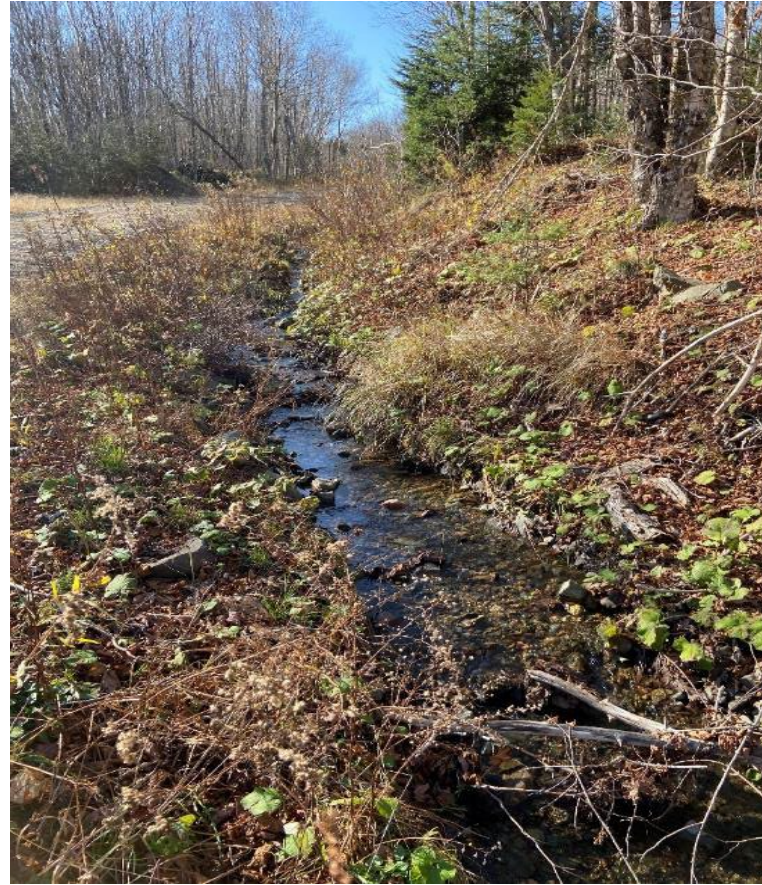
Photo 2: Feature 1 (Road side ditch connected to watercourse)
