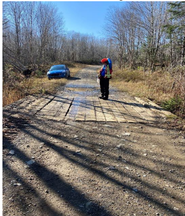
Photo 4: Feature 2 (bridge/crossing over watercourse)
