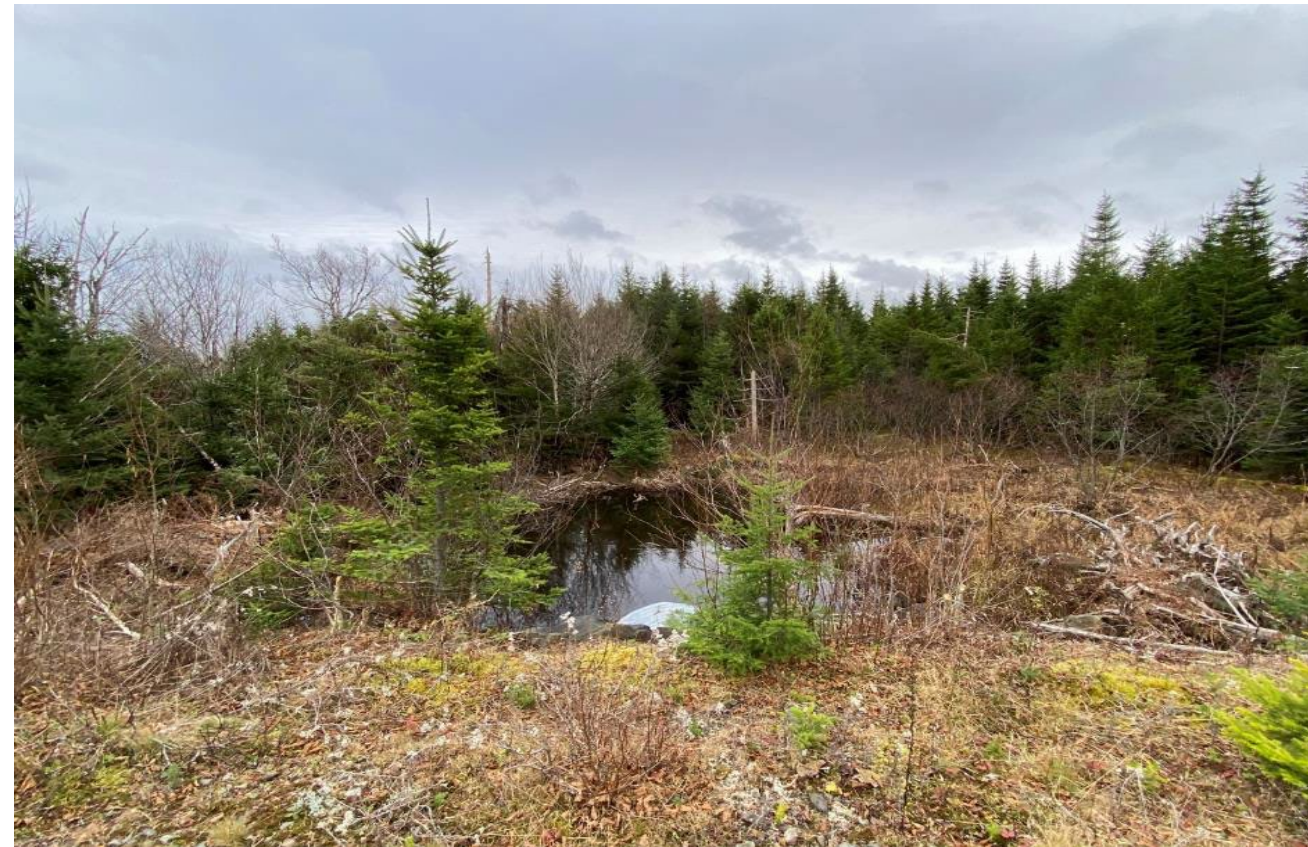
Photo 2: Downstream at Crossing Location (downstream of culvert)
