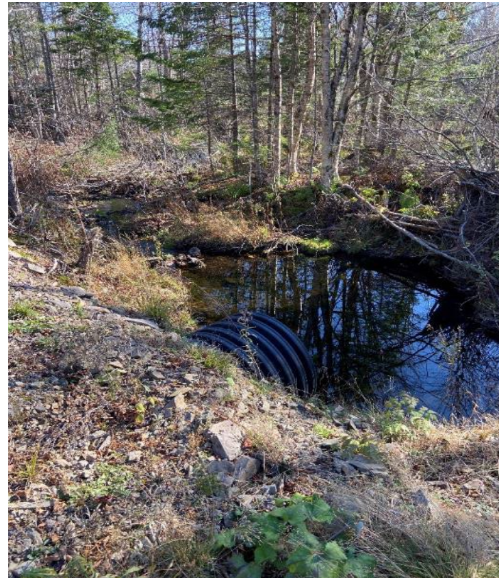
Photo 2: Downstream at Crossing Location
