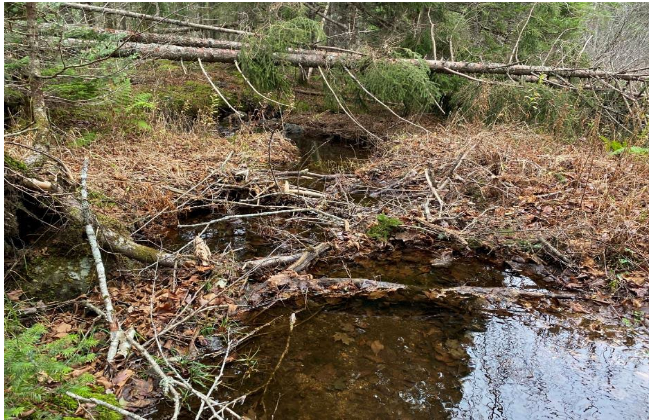
Photo 1: Upstream at Crossing Location
