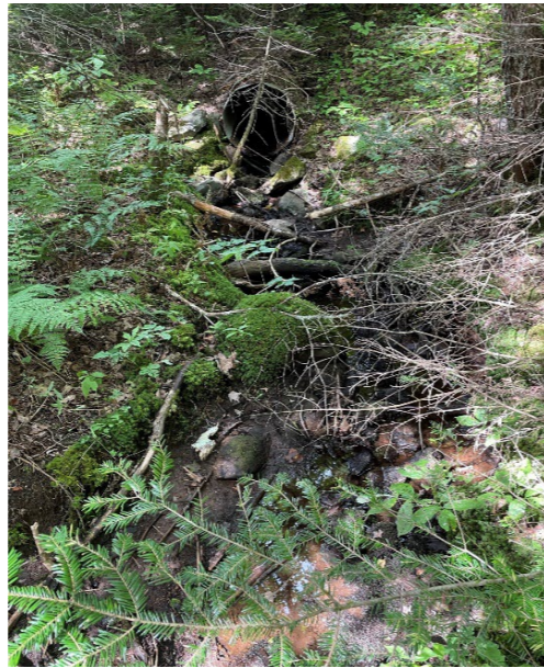
Photo 1: Upstream culvert at approximate crossing location.
