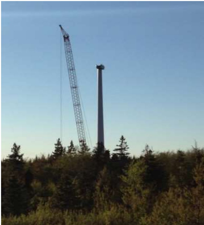
Figure 6.5 Turbine Tower Erected with Crane Ready to Hoist Blade Assembly
