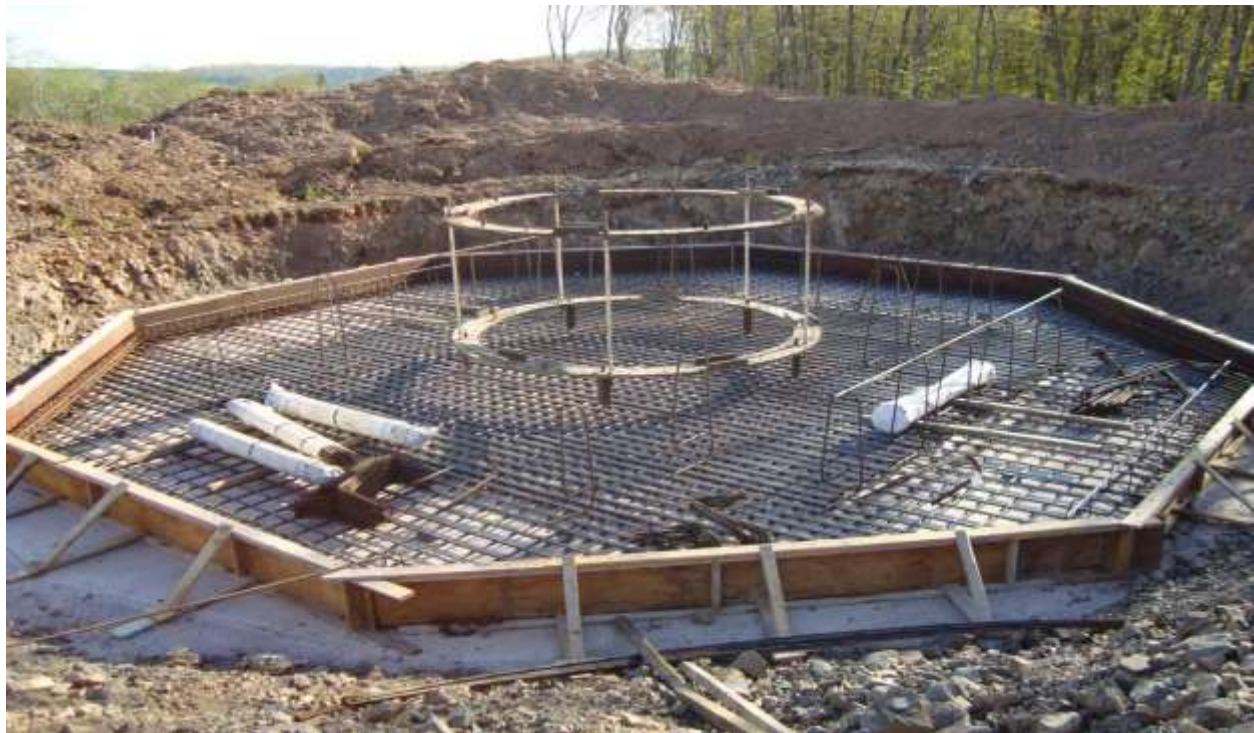
Figure 6.2 Foundation Partially Complete with Frames and Rebar in View
