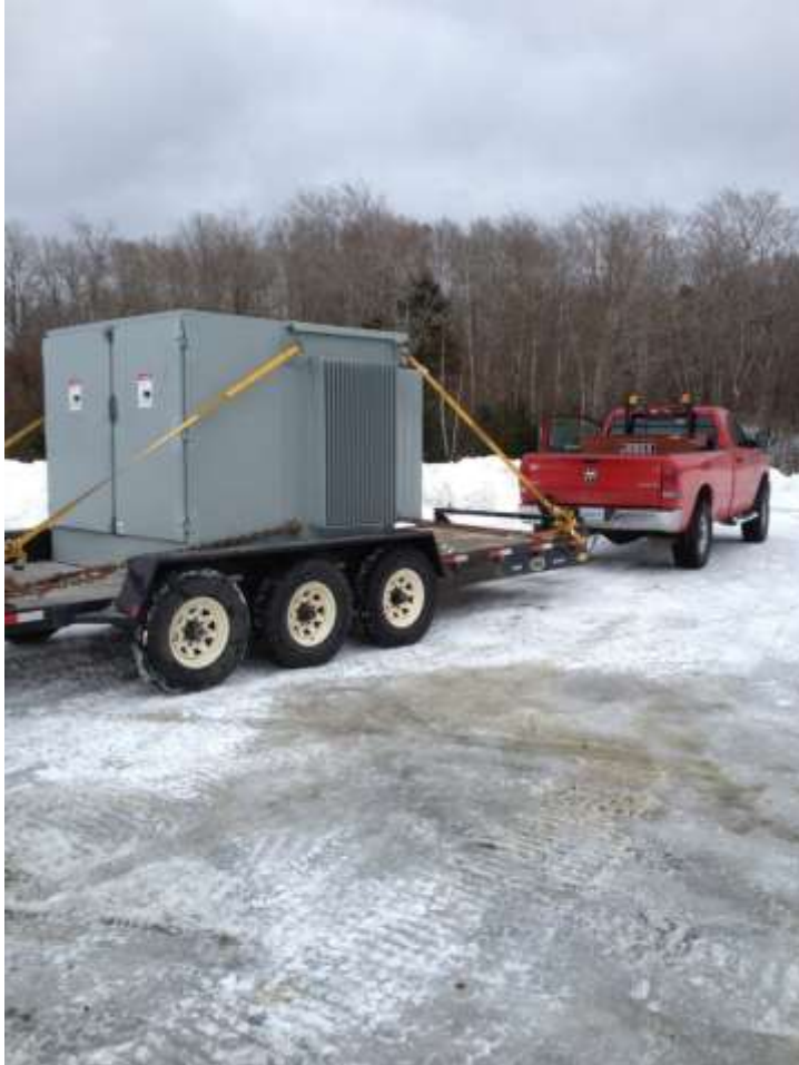
Figure 2.5 Pad mounted step-up transformer to convert 690V from turbines to collector lines.
