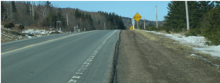
Photo 2.12 - Looking north on Route 344 on the approach to the turn just south of Highway 104. Note that the TURN sign is hidden by the crest.
