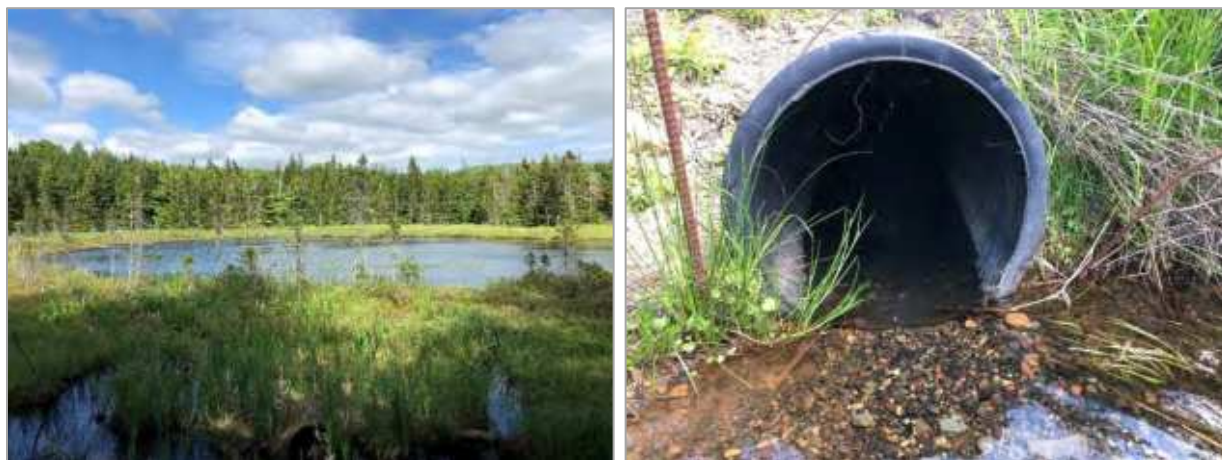
Figure 21. Westernmost pond (left) and exit culvert under MacIntyre Road, June 15, 2021.
