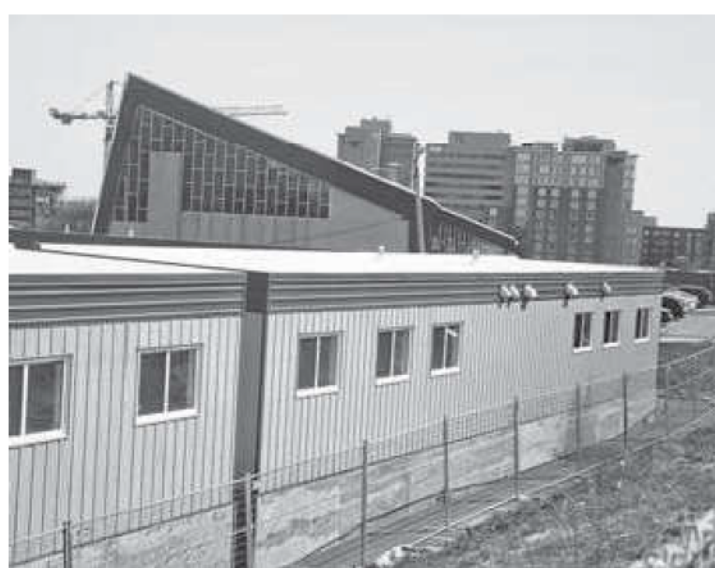
The emergency modular housing units behind Halifax's Centennial Pool are seen on Tuesday, April 26, 2022. RYAN TAPLIN ■ THE CHRONICLE HERALD
