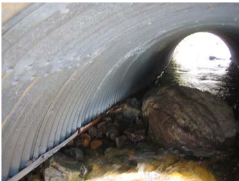
The existing open-bottom allows for potential fish habitat
