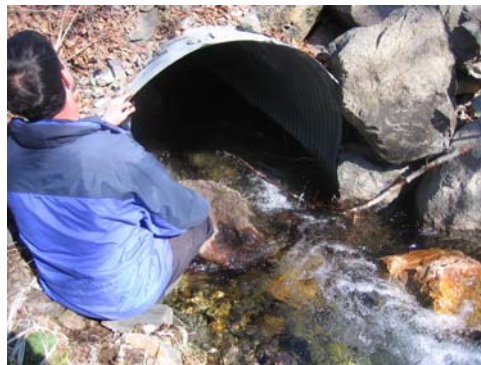
Existing CMP box culvert (Culvert A) over a tributary of the Waugh River to be extended
