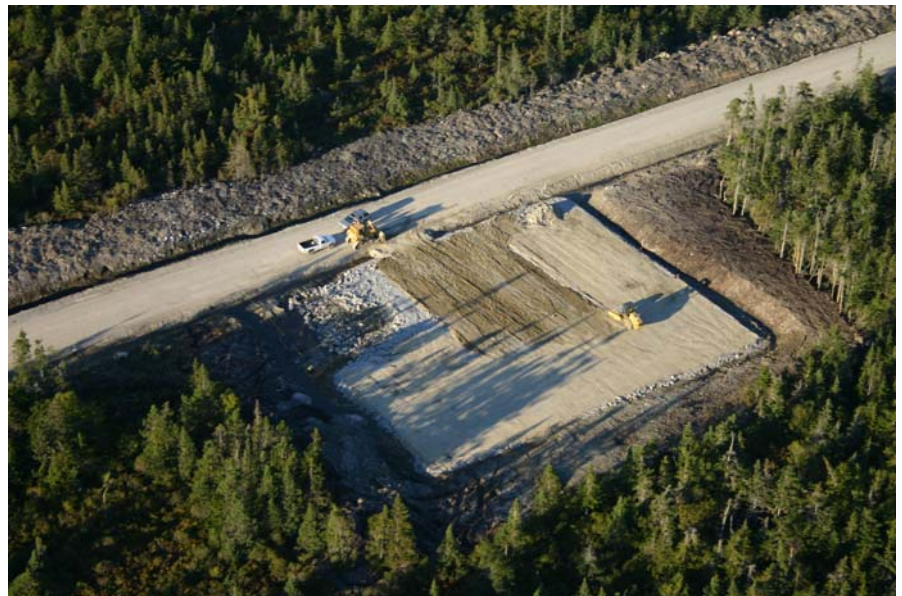
Preparation of Typical Crane Pad and Lay Down Area at Pubnico Point Wind Farm
