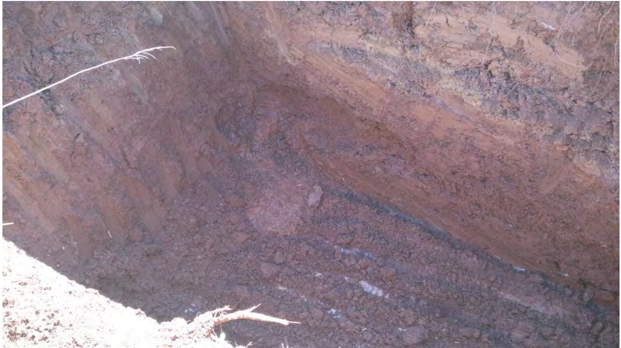
Photograph 1: Test Pit 1. May 9, 2013.
