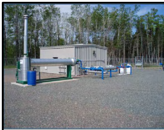
“Example of Heritage Gas High Pressure Reducing Station”
