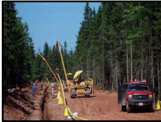
"Typical Heritage Gas pipeline under construction"
