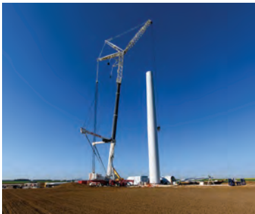
Building the tower
