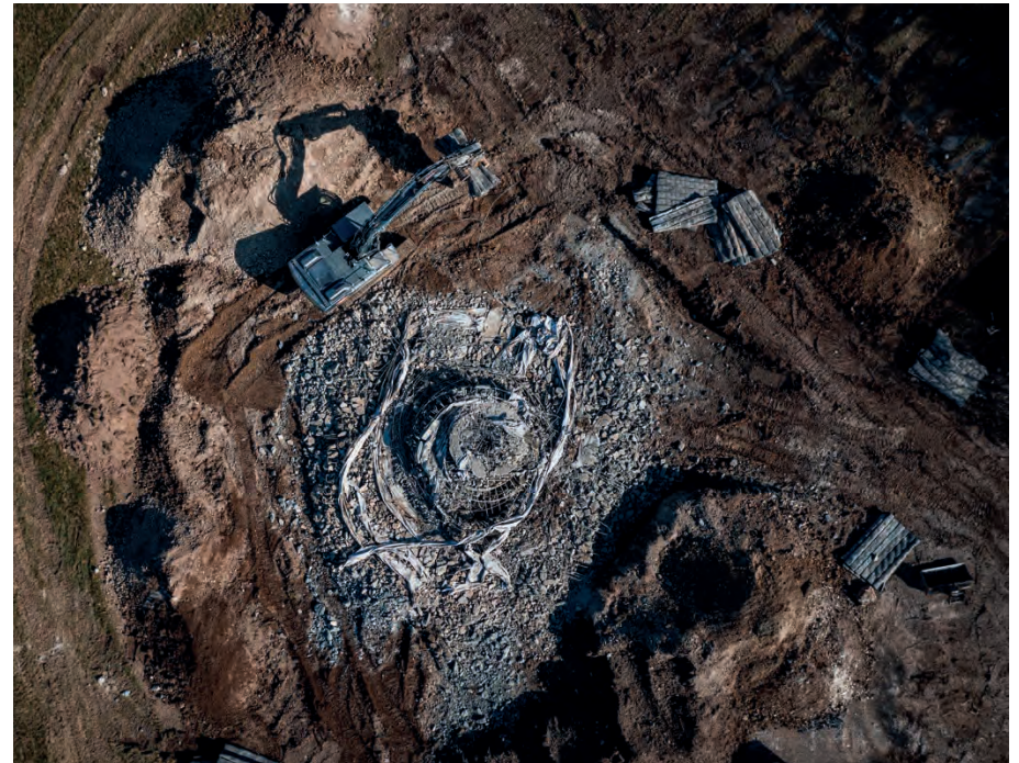
Deconstruction of foundation
