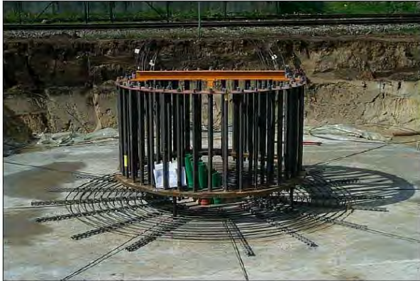
Erected and adjusted bolt cage
