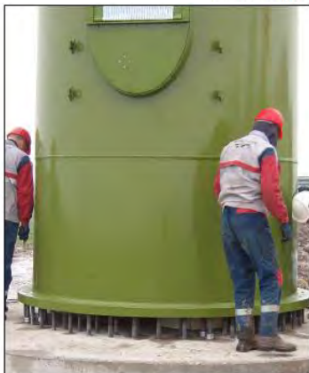
Placing the bottom tower segment
