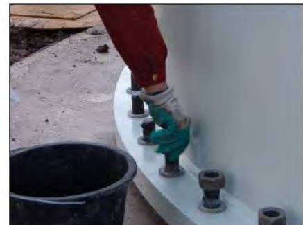
Bolting the tower segment
