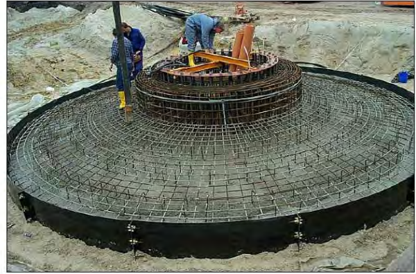
Foundation reinforcement with integrated bolt cage
