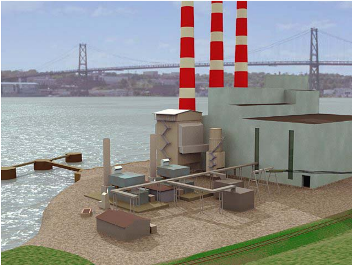
Figure 1: Sketch of Tufts Cove Generating Station – showing existing and proposed Combustion Turbine units. TUC 5 is the rightmost of the two smaller units next to the powerhouse for Units 1-3 at the Tufts Cove Generating Station.
