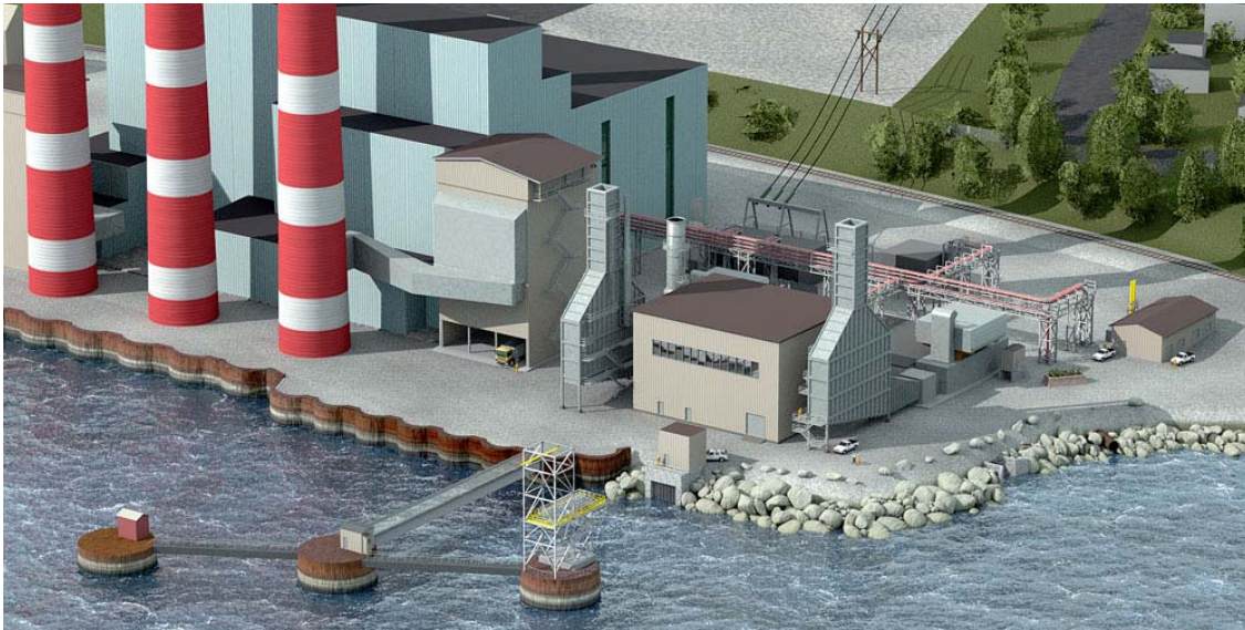
Figure 3 Sketch of Tufts Cove Generating Station – showing existing CT Units 4 and 5 and proposed TUC 6 powerhouse adjacent to powerhouse for Units 1-3
