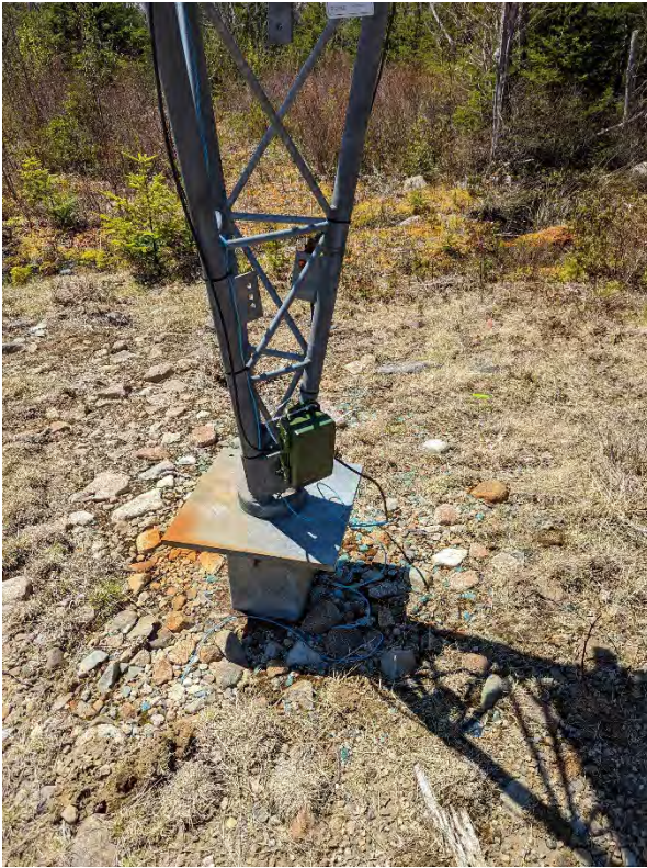
Photo 1: Installation of Bat 1
