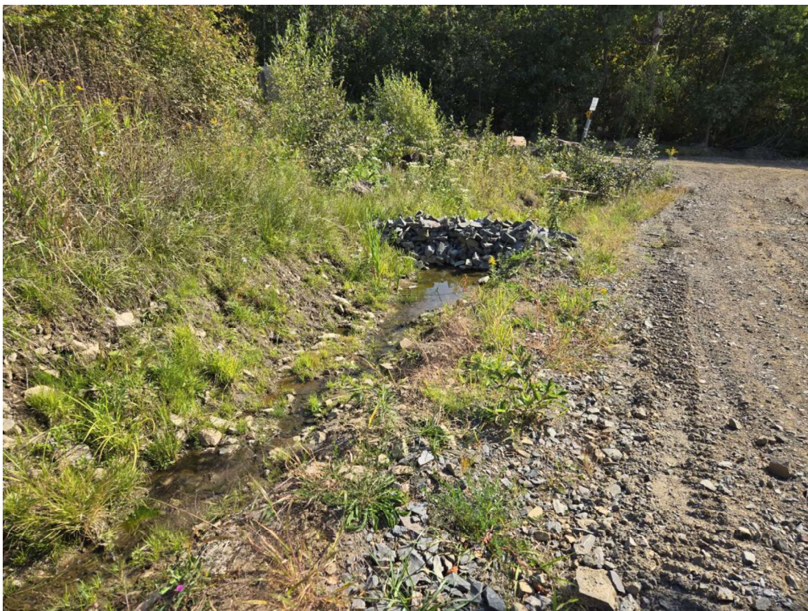
Figure 6.4. Representative view of primary drainage ditch beside the main Site access (September 16, 2025).
