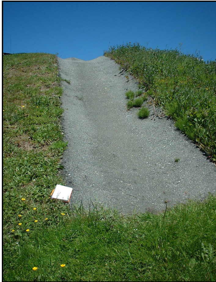
Photo 8 Asphalt Apron at Kent Building Supplies
