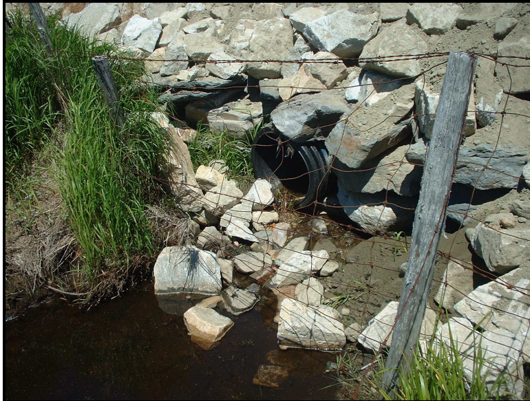
Photo 2 Downstream Portion of Culvert on Dirt Road
