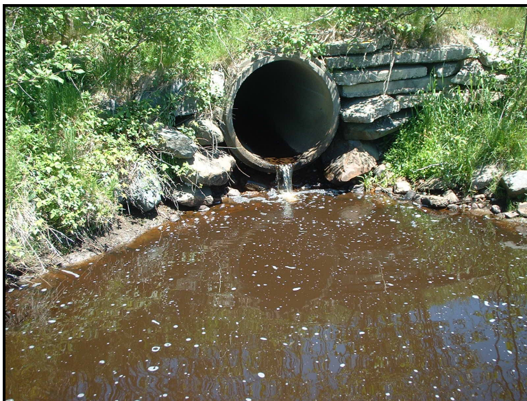
Photo 9 Perched Culvert Downstream Side of Starrs Road
