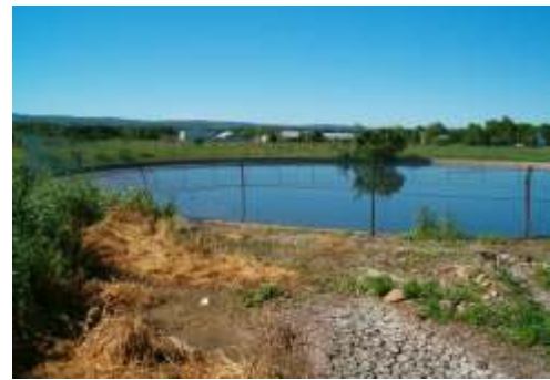
Non-earthen Liquid Manure Storage
