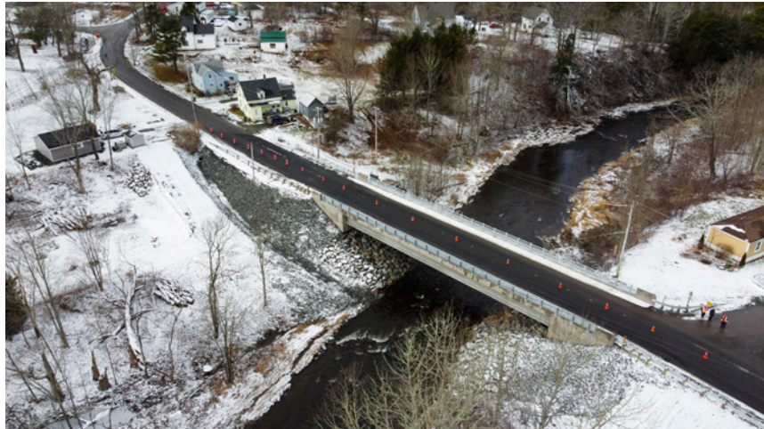
Eureka Mills Bridge
