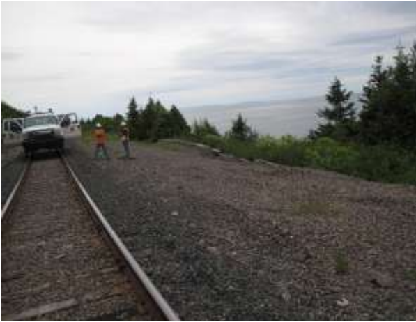
Photo 12 – Mile 3.0 : Non Subsidized Line Easterly Looking Westerly June 18, 2014
