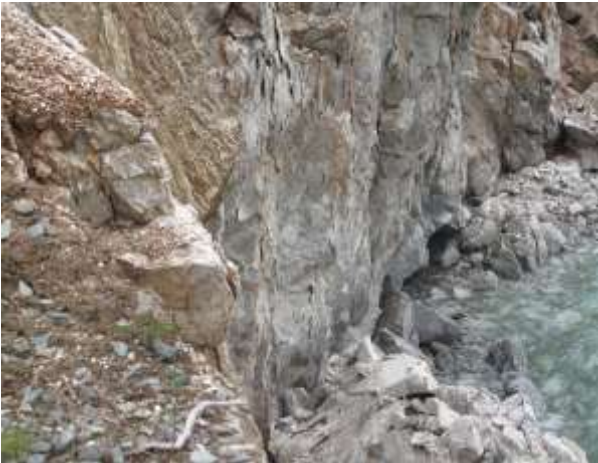
Photo 25 – Mile 54.6: Subsidized Line Close Up of Toe of Cliff June 18, 2014
