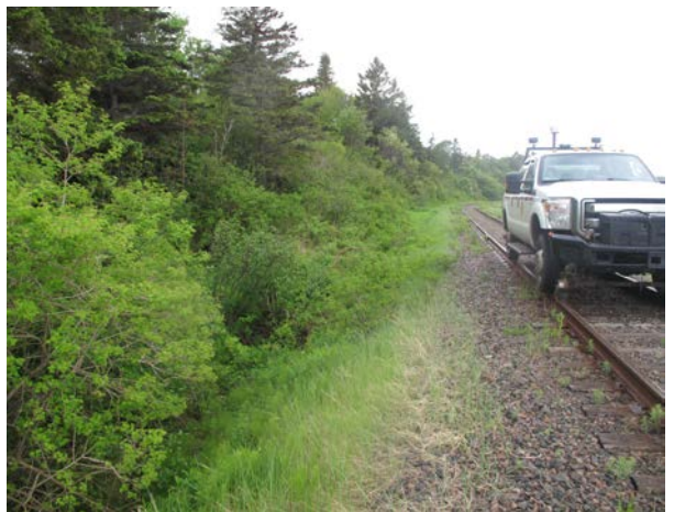
Photo #64 - Mile 58.8: Subsidized Line East Looking Westerly, South Side of Rail
