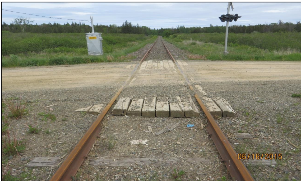
M.P. 52.08 - ROAD CROSSING – FLASHING LIGHTS Gravel roadway approaches and wood planks
