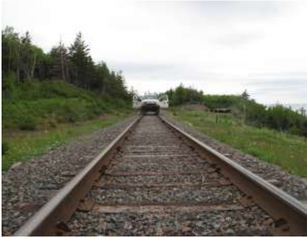
Photo 1 – Mile 2.8: Non Subsidized Line Easterly Looking Westerly June 18, 2014
