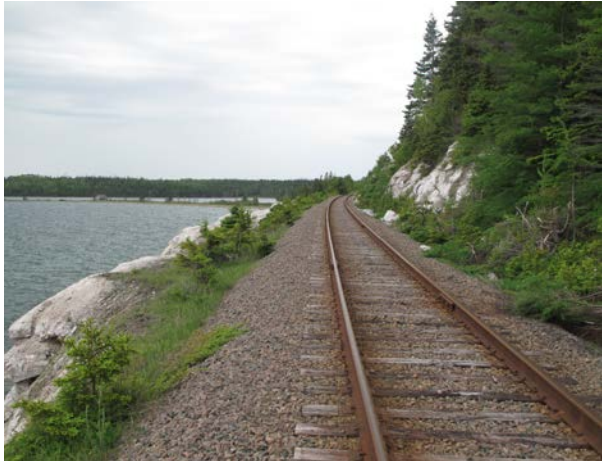
Photo #53 - Mile 53.8: Subsidized Line East looking West - Crest of Embankment
