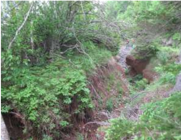
Photo 43 – Mile 68.3: Subsidized Line North Looking South: Slope Movement
