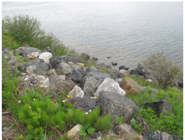
Photo #62 - Mile 58.8: Subsidized Line Location Remediated East of Subject Slope
