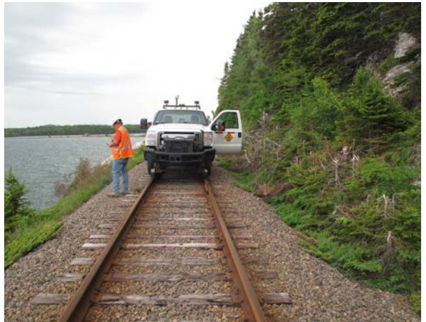
Photo #56 - Mile 53.8: Subsidized Line East Looking Westerly
