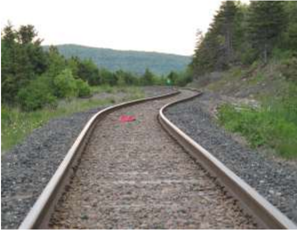
Photo 7 – Mile 2.9: Non Subsidized Line Westerly Looking Easterly: Line Realignment June 18, 2014
