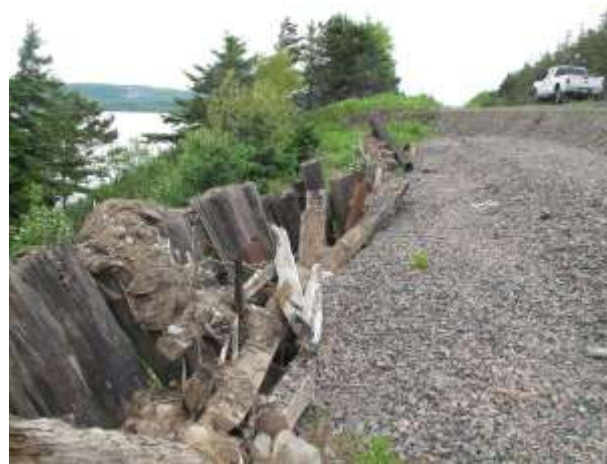
Photo 17 – Mile 3.0: Non Subsidized Line Middle of Slope/Crest of Retaining Wall June 18, 2014
