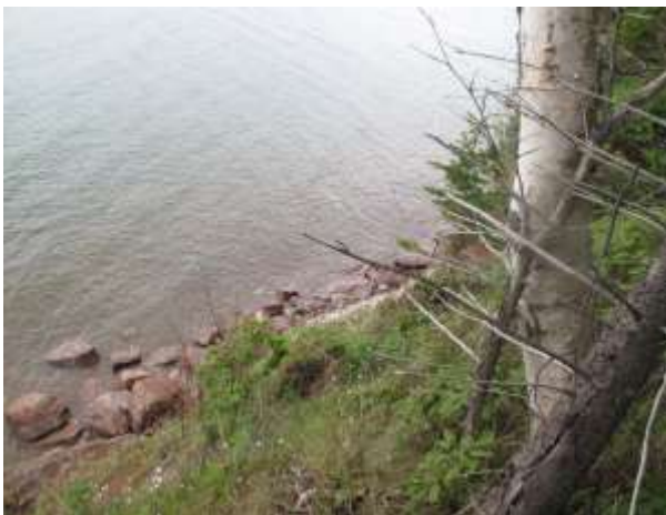
Photo 45 – Mile 68.3: Subsidized Line Conditions at Toe of Slope
