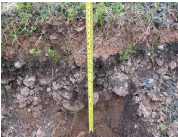
Photo 39 – Mile 60.1: Subsidized Line Crest of Slope Consisting of Fill June 18, 2014
