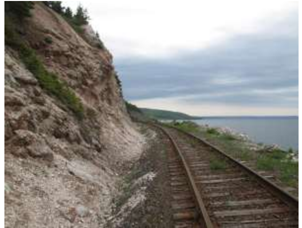
Photo 26 – Mile 54.6: Subsidized Line South Side of Line June 8, 2014
