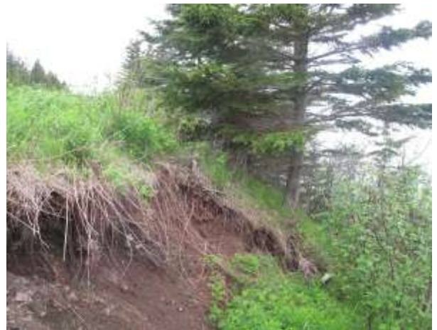
Photo 40 – Mile 60.1: Subsidized Line Close Up of Sloughing Near Crest of Slope June 18, 2014
