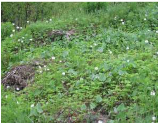
Photo 5 – Mile 2.8: Non Subsidized Line Toe of Slope on North Side of Line June 18, 2014
