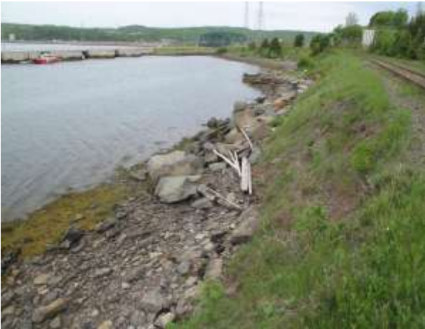
Photo 20 – Mile 8.5: Non Subsidized Line South Side of Line: Toe of Slope
