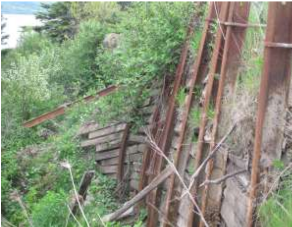
Photo 16 – Mile 3.0: Non Subsidized Line Middle of Slope/Toe of Retaining Wall June 18, 2014
