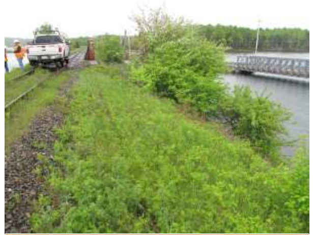
Photo 48 – Mile 103.3: Subsidized Line North Looking Southerly: West Side of Line June 18, 2014
