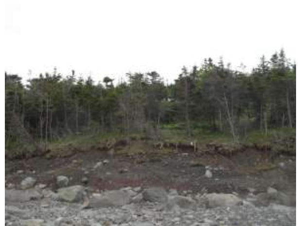
Photo 6 – Mile 2.8: Non Subsidized Line North Looking South: Toe of Slope June 18, 2014
