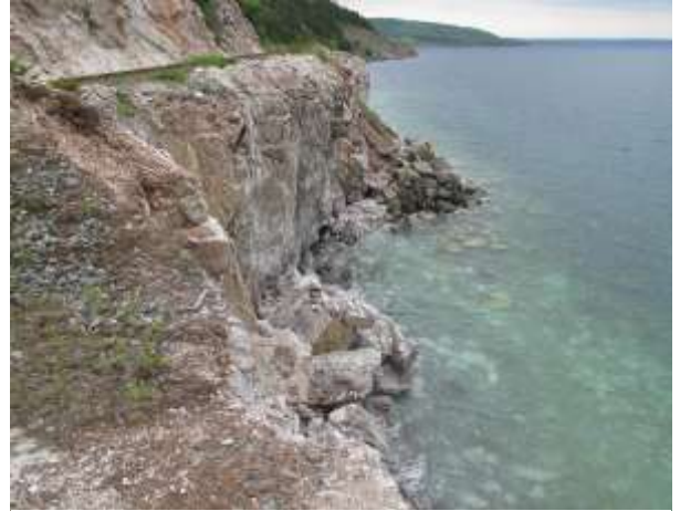
Photo 24 – Mile 54.6: Subsidized Line Undermining at Toe of Cliff June 18, 2014
