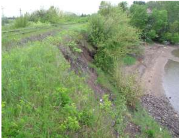
Photo 49 – Mile 103.3: Subsidized Line North Looking South: East Side of Line: June 18, 2014
