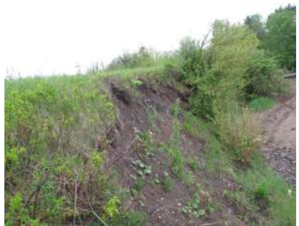
Photo 52 – Mile 103.3: Subsidized Line Close Up of Soughing at Crest of Slope June 18, 2014
