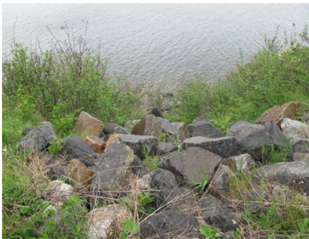
Photo #63 - Mile 57.0: Subsidized Line Location Remediated West of Subject Slope
