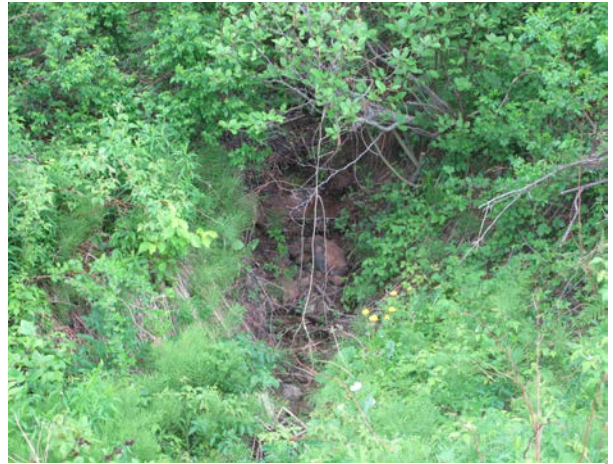
Photo #60 - Mile 57.0: Subsidized Line Surficial Sloughing
