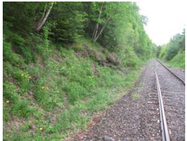
Photo 46 – Mile 68.3: Subsidized Line South Side of Line
