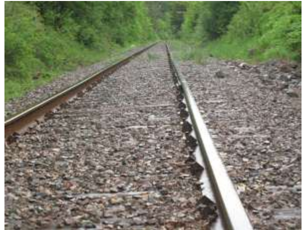
Photo 44 – Mile 68.3: Subsidized Line Easterly Looking Westerly: Close Up of Line
