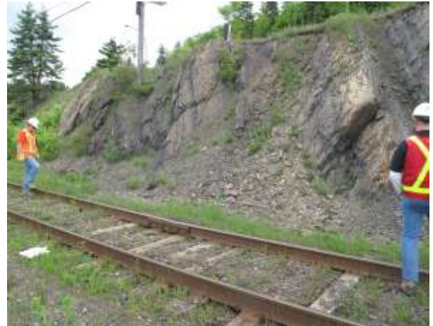
Photo 21 – Mile 8.5: Non Subsidized Line North Side of Line: Bedrock Outcrop
