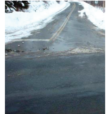
Road where anti-icing was used.
