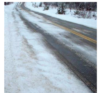
Road where anti-icing was not used.
