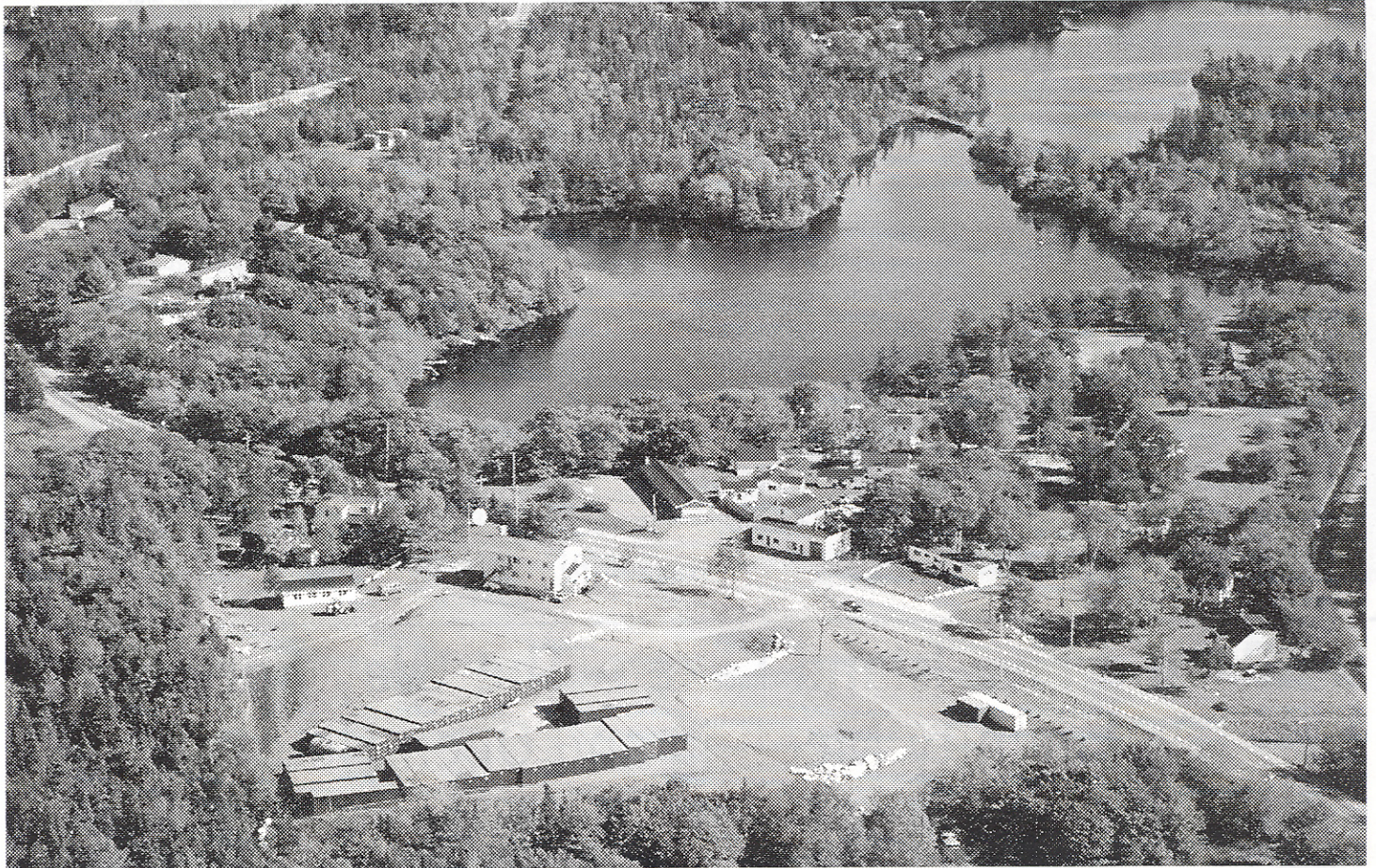
Aerial view of the site, showing the storage containers (soon to be removed) and the gravel cap over the buried wastes.
