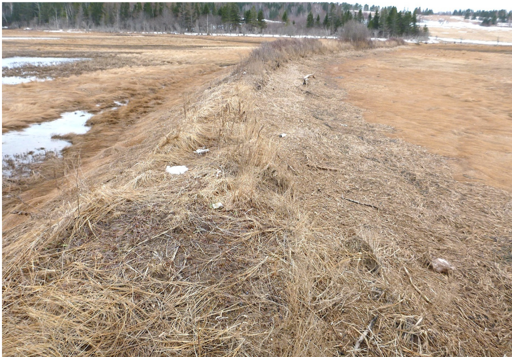
Figure 64 Vegetative material and large woody debris along downstream side of dyke at CHV. The dyke itself has suffered much erosion and subsidence over the past several years. Photograph by T. Bowron, 15 March 2011.
