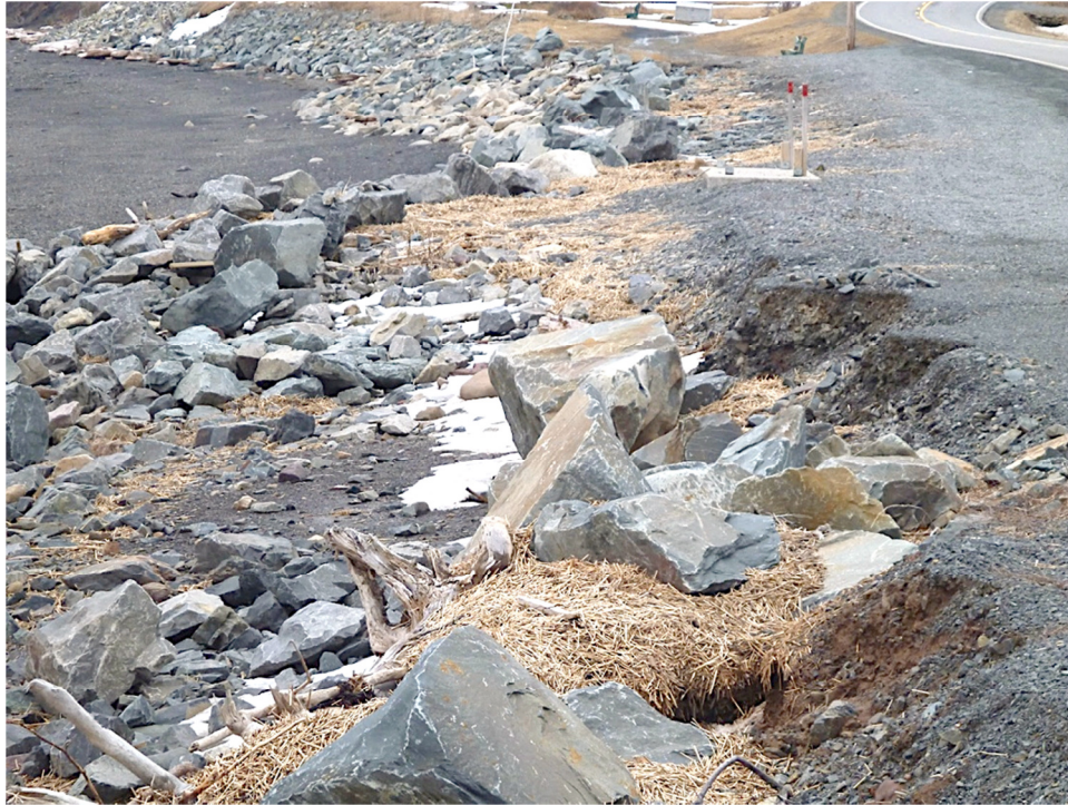
Figure 67 Loss of armour stone and erosion of fill along seaward side of causeway. Photograph taken at mid-causeway looking north away from culvert. Photograph by T. Bowron, 6 March 2013.
