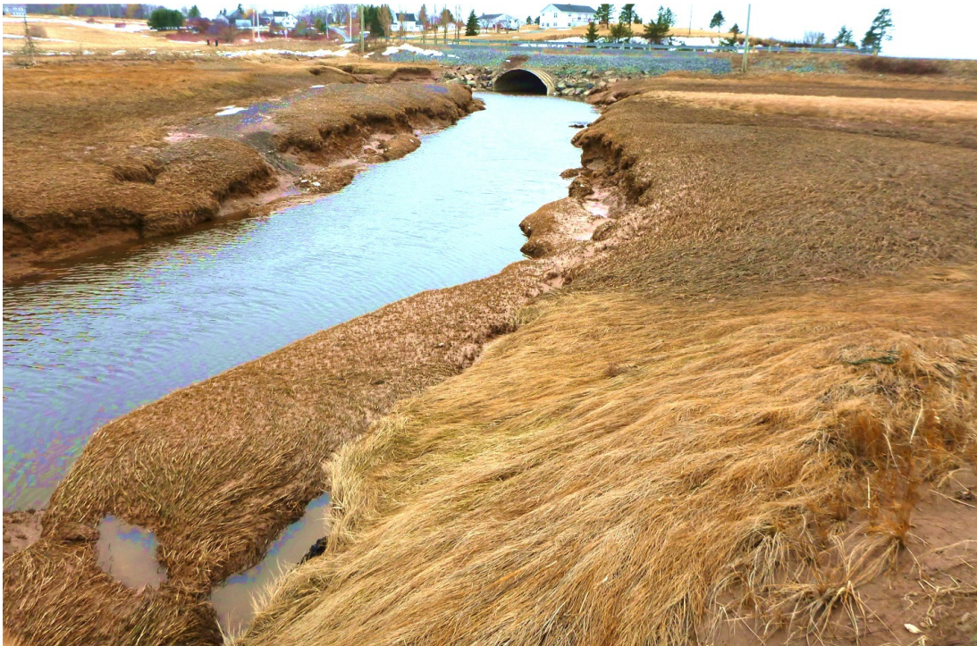
Figure 62 Bank slumping and erosion along the main channel at the toe of the dyke. Photograph by T. Bowron, 15 March 2011.
