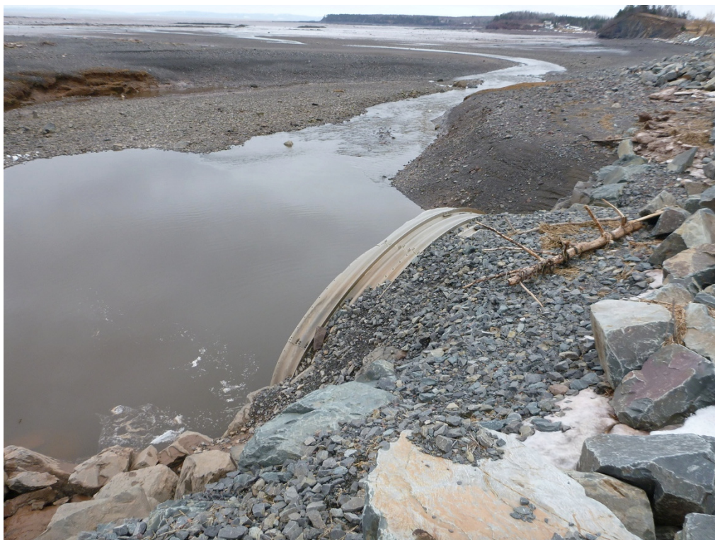
Figure 8 Downstream end of culvert, coastal berm and channel.
