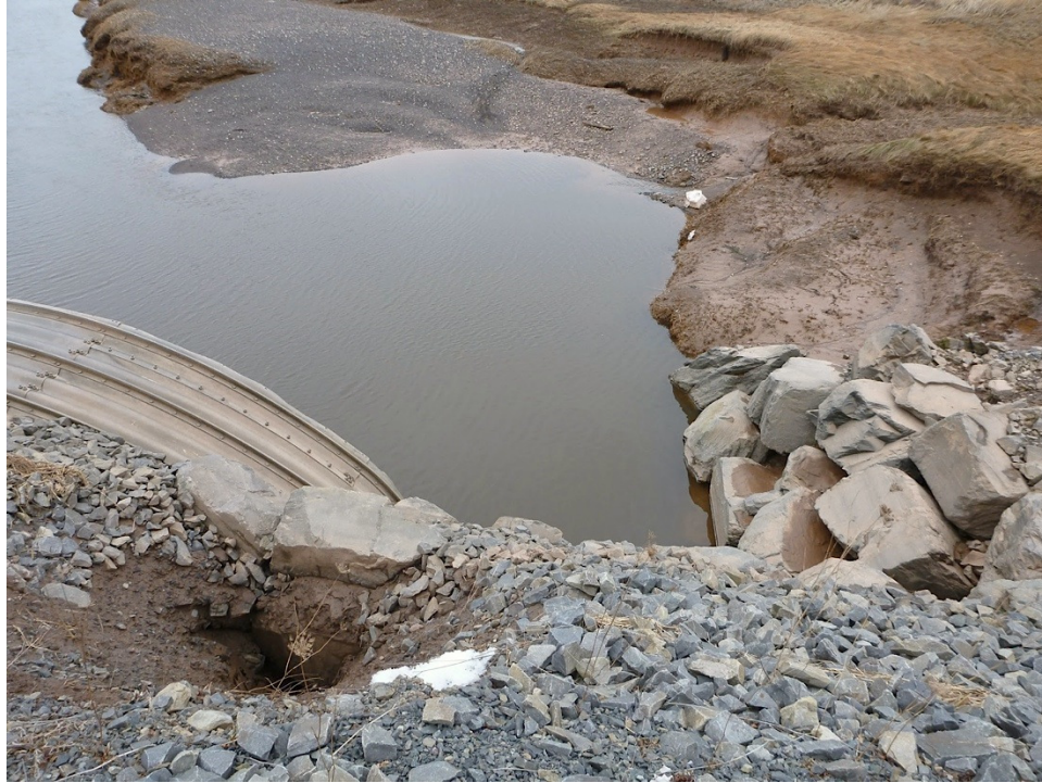
Figure 63 Erosion around the upstream end of the culvert. Photograph by T. Bowron, 6 March 2013 (NB: NSTIR added additional armour stone in Summer 2013).
