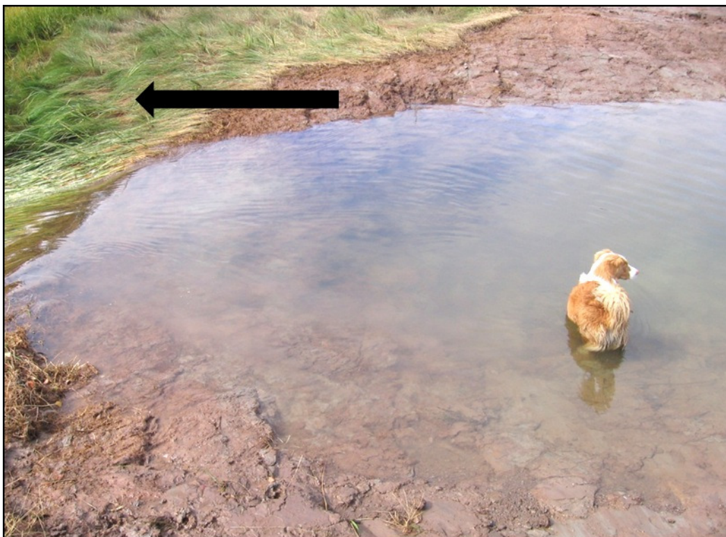
Figure 5: The central tide channel (“main channel”), constructed by digging an approximate 2 m wide x 0.5 m deep trench. Black arrow is pointing towards river. Photograph by T. Bowron, fall 2005.
