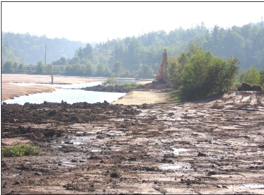
Figure 4: Earthworks at WAL in fall of 2005 showing partial infilling of borrow pit.
